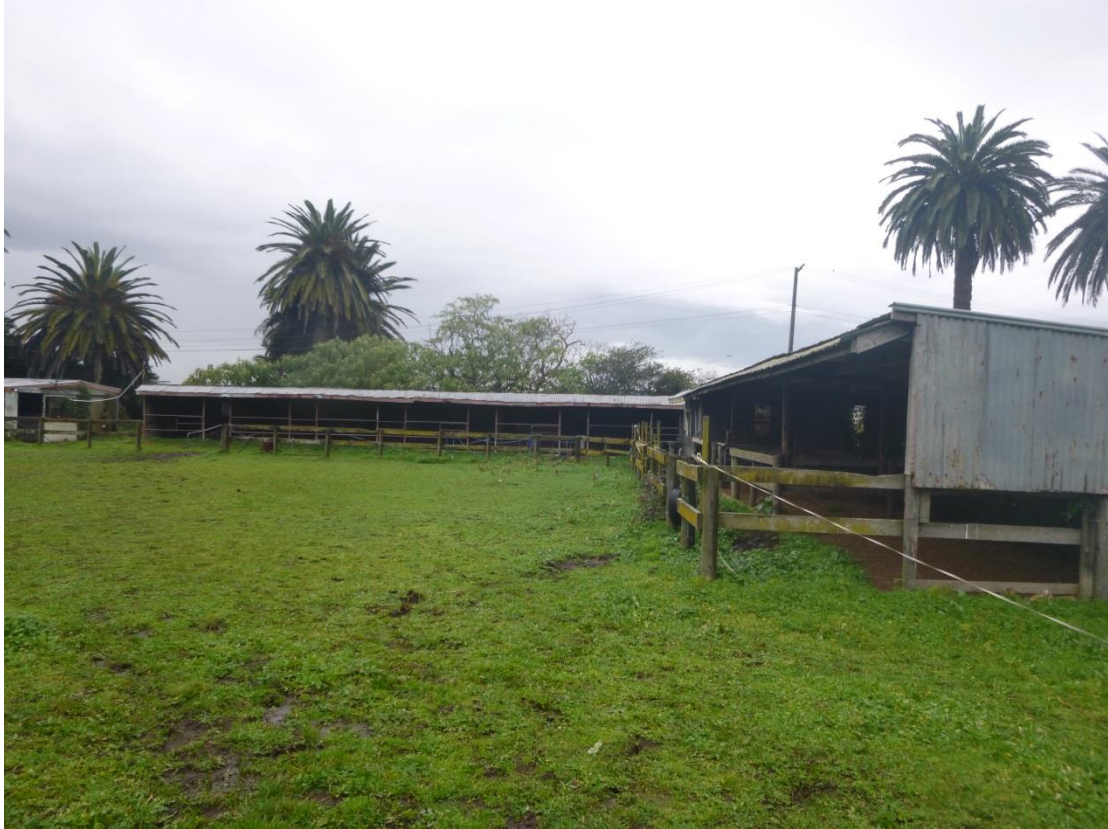
Photograph 8: Stables 3 and 4 at the north western property boundary (looking west).
